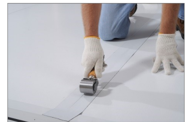
Roll firmly with a hand roller.
