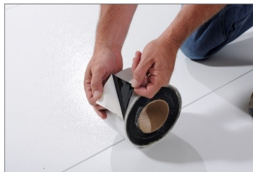
Peel back the release liner.
