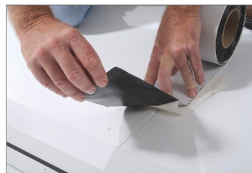
Center over the panel seam.
